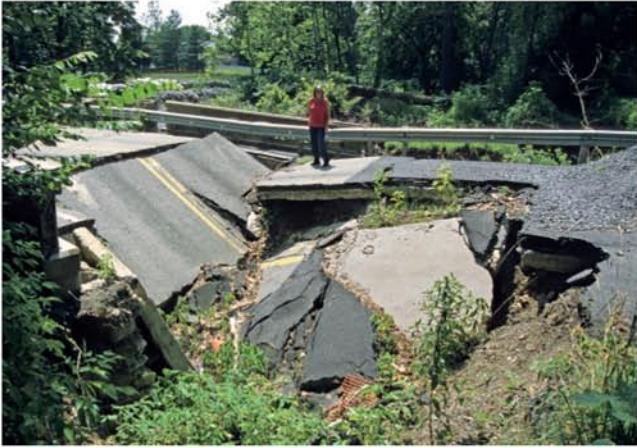
Fig. 6. The approach to the Tatamy bridge, destroyed by active sinkholes.
