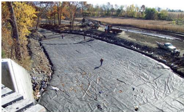
Fig. 5. Installing the liner along the creek bed downstream of Stockertown Quarry (photo: Brookwood Group).
