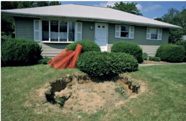
Fig. 2. A small subsidence sinkhole that was a dropout in the front lawn of a house in Pennsylvania affected by de-watering of a nearby quarry.
