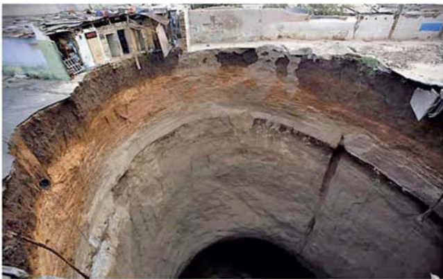
Fig. 11. Weak pyroclastic sediments that are prone to piping failure, exposed in the new sinkhole in Guatemala City.
