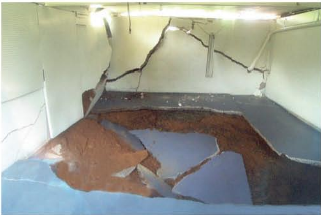
Fig. 7. The basement floor of 29 Babbling Brook Road, which collapsed into an expanding group of subsidence sinkholes (photo: Brookwood Group).
